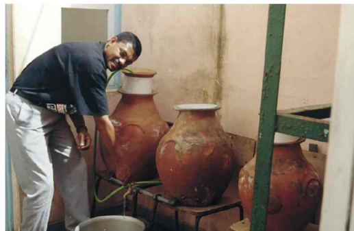
Carlos Monteiro by the sand filters for the fog water collection system on Santiago Island in the Cape Verde Islands.
