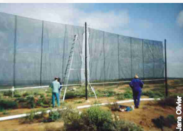
Johann van Heerden and two workers installing the fog collectors at Lepelfontein, South Africa.
