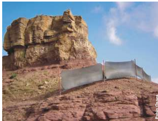
Large fog collectors were built to provide water for the small village of Shamsan, Yemen.
