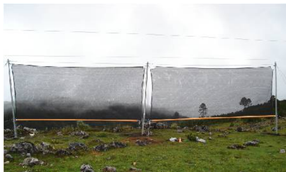
Two of the four finished fog collectors in Tojquia.
