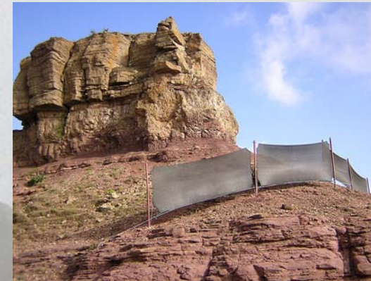
Each fog collector is 6 m high and 10 m long.
