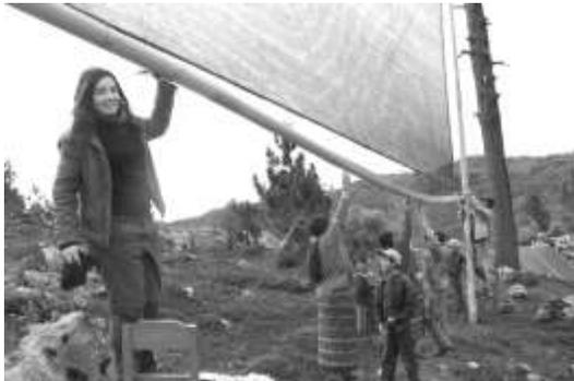
Photograph 2: Installing the trough on a fog collector, with the help of the entire family.
